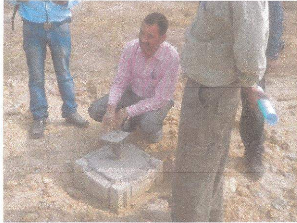
Fig. 14: Monitoring stations were installed with 1.0 m long pipes and masonry pillars
