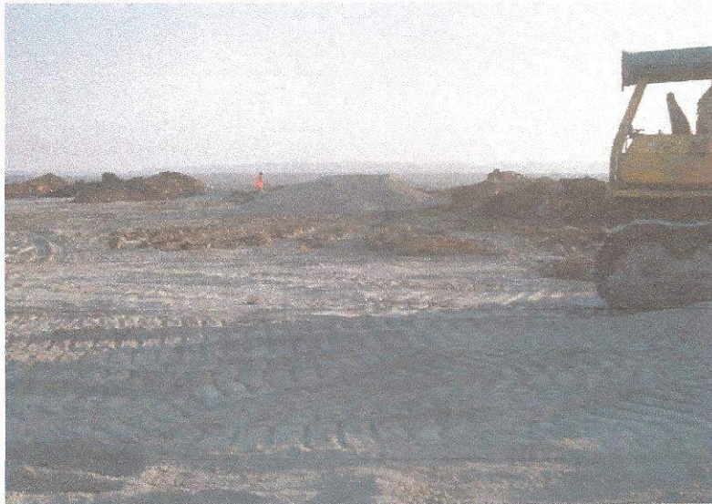
Fig. 2c: Dozing of fly ash and OB material at the dump site
