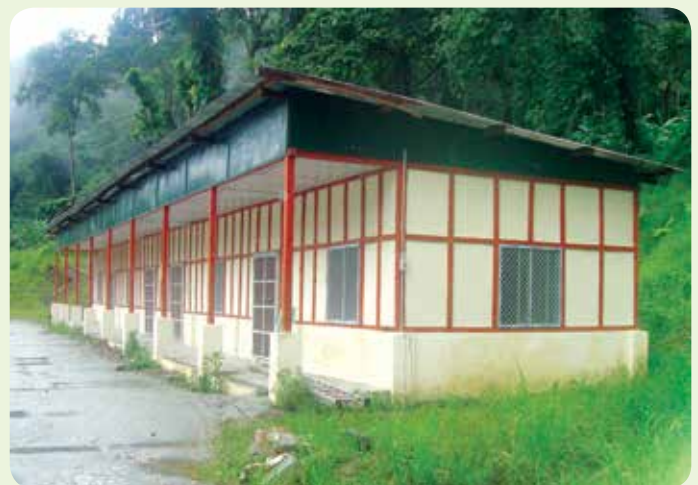
Construction of Semi Permanent Type Building
