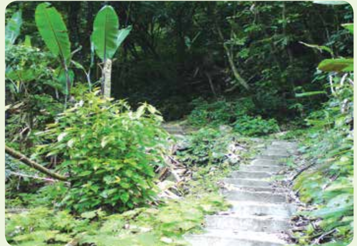
Construction of Cement Concrete Steps
