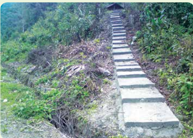
Construction of Cement Concrete Steps
