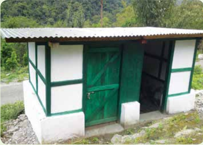
Construction of Toilet at Punli (Dri) L.P School
