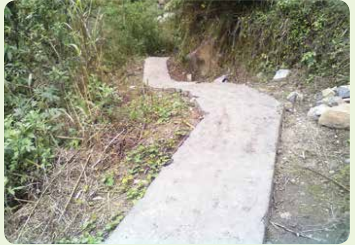
Construction of Cement Concrete Foot Way
