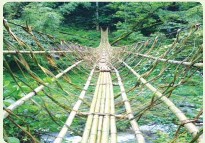
20 Nos. hanging bridge repaired & renovated
