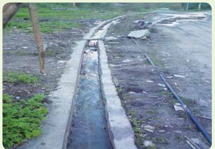
Construction of Cement Concrete Drain
