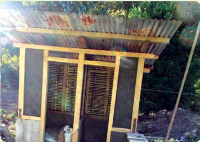
Construction of toilet at Punli (Talo) village
